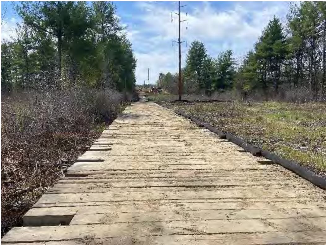
Fig 20: Access road swept and maintained through wetland DW58. Viewing south. (05-06-20).
