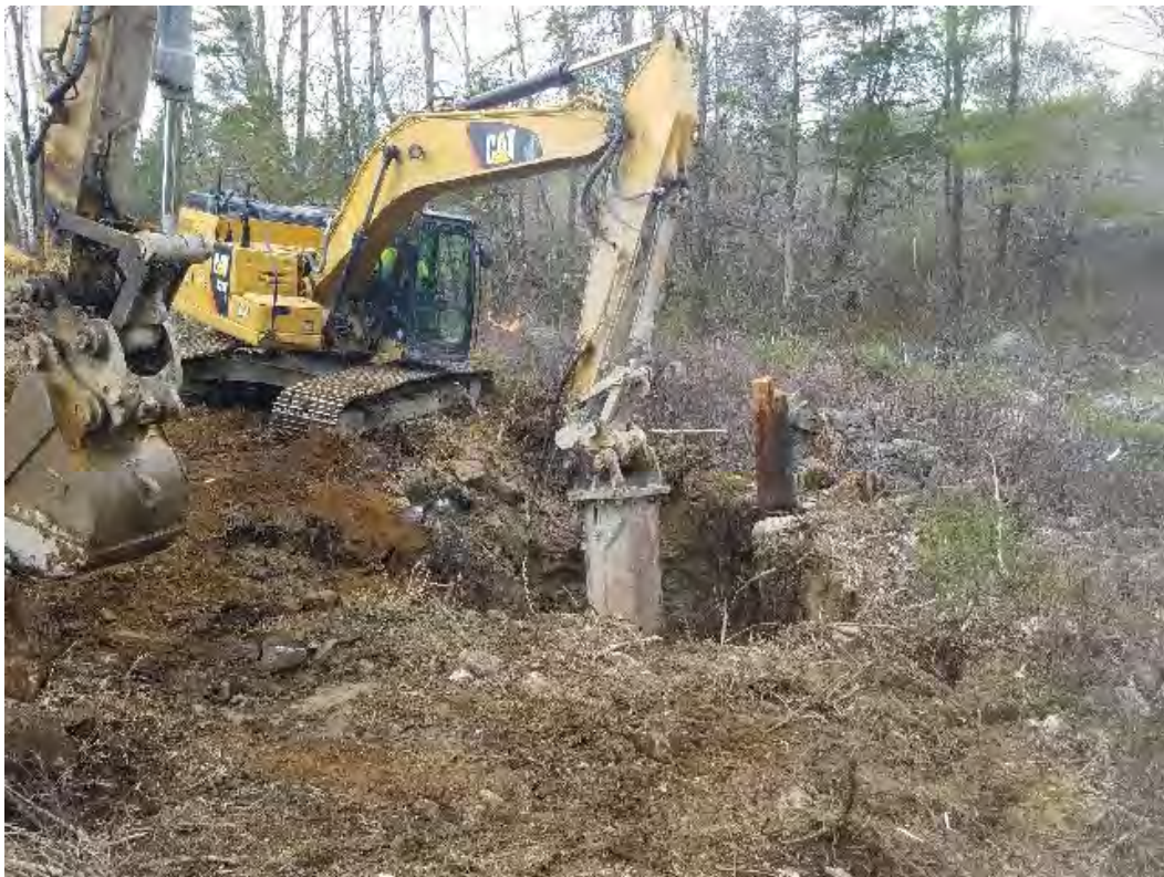
Fig 10: Hammering ledge at Str. 45. Viewing west. (05-04-20).
