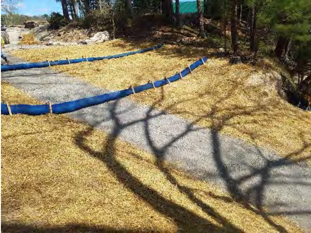
Fig 15: Installing BMPs on slope at Gundalow landing/east side of the Bay. Viewing southeast. (05-05-20).
