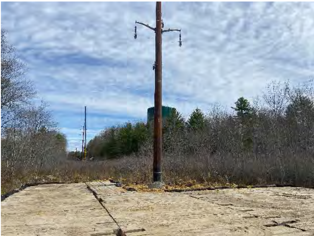
Fig 18: Str. 35 pole set. Viewing north. (05-06-20).
