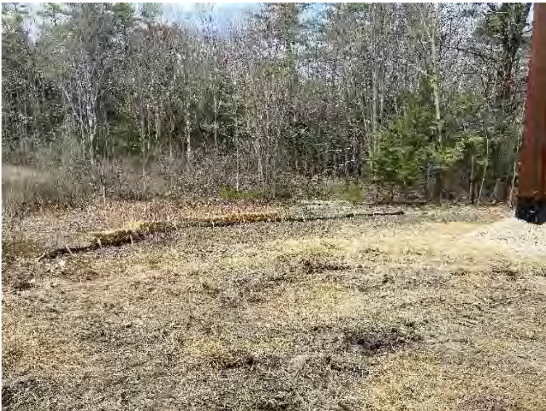
Fig 22: Combined berm installed downslope of Str. 82. Viewing north. (05-06-20).
