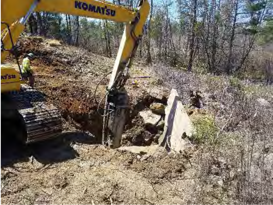
Fig 17: Hammering ledge at Str. 45. Viewing west. (05-05-20).
