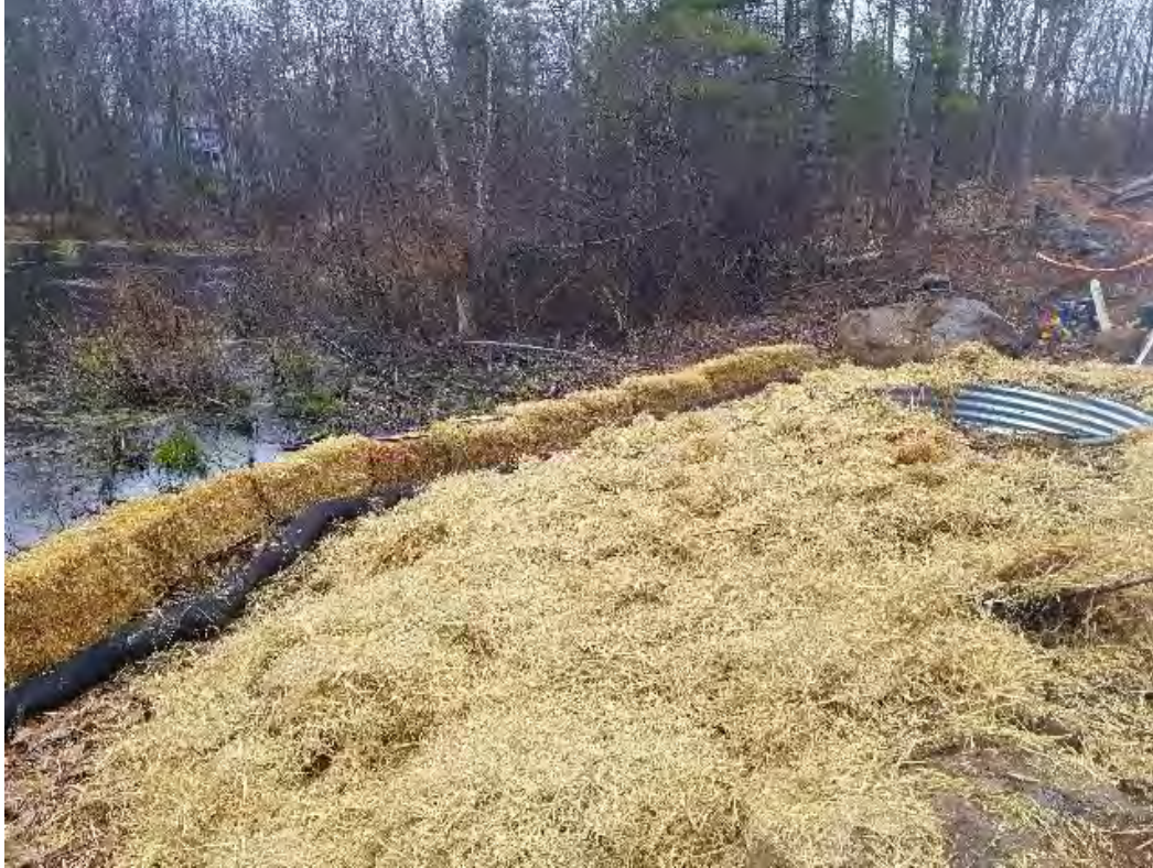
Fig 3: Str. 34 foundation can set. Viewing northwest. (04-30-20).
