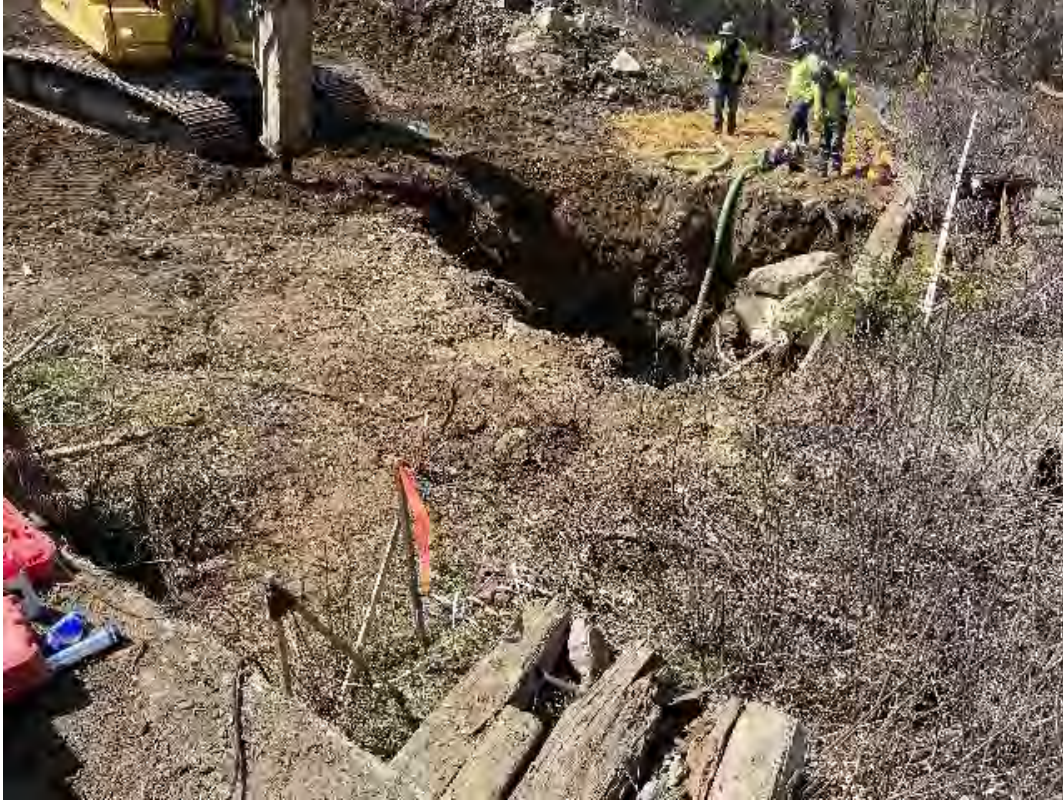
Fig 19: Pumping water out of hole at Str. 45. Viewing west. (05-06-20).
